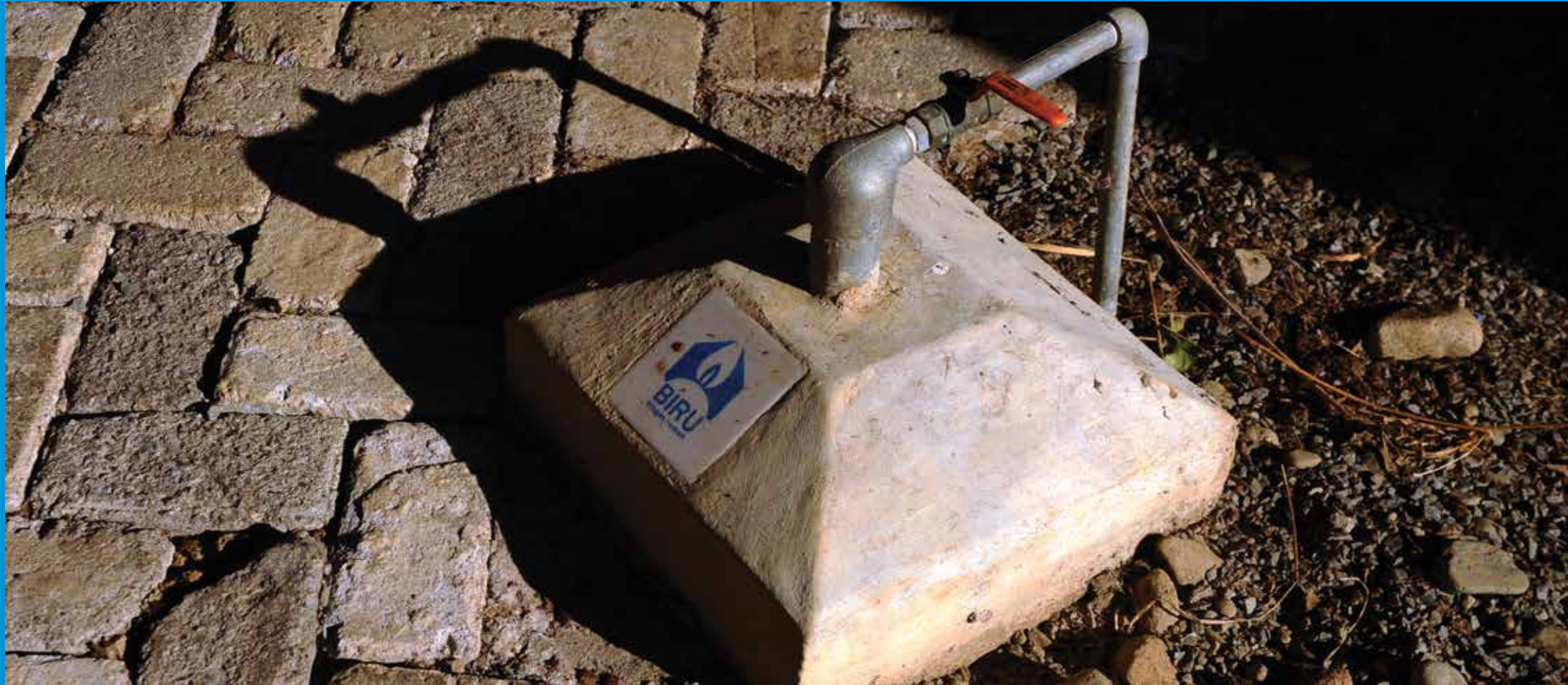
Pipa gas utama reaktor biogas / Biogas digester main valve
