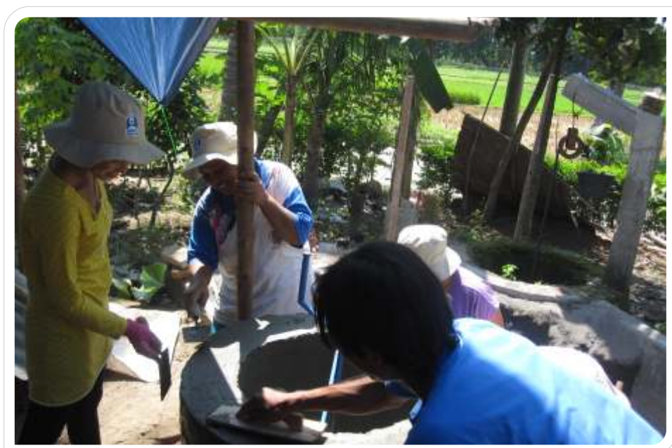
Image 13: Female masons work on bio-digester construction in Central Java, 2012.
