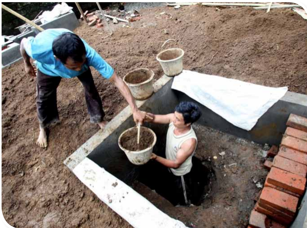
Biodigester construction in Bali
