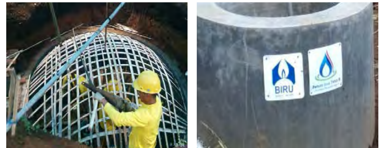
Picture 10: Construction of biodigester in partnership with PJT II at Padamukti - West Java
